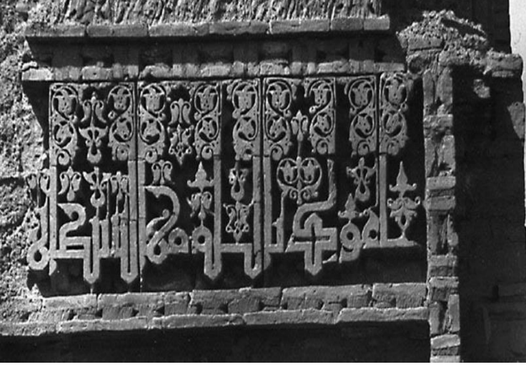
Hargird Medresesi ( http://www.selcuklumiirasi.com/architecture-detail/hargird-nizamiye-medresesi )
